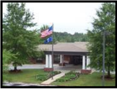
Richard M. Campbell Veterans' Nursing Home - a 220-bed skilled nursing care facility for Veterans in Anderson.
